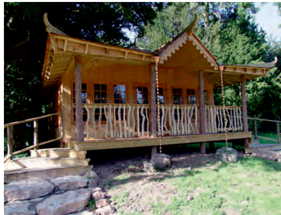
Figure 4: The new teahouse built on the elevated sloping ground.
