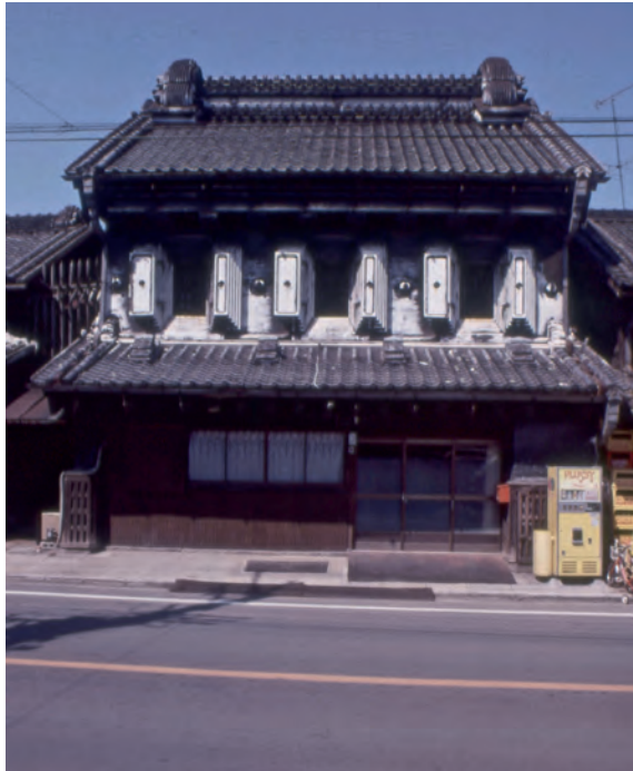
The walls and window openings resist the ravages of fire.
