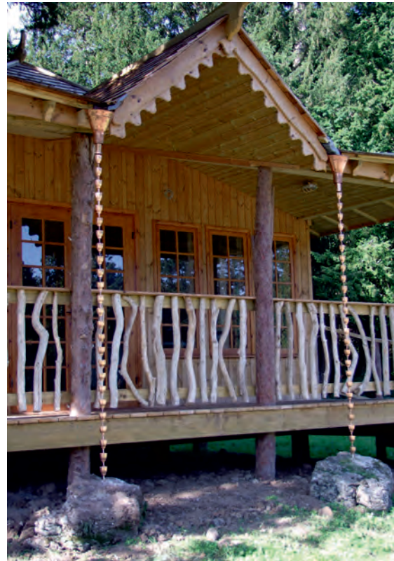
Figure 5: Cedar shingle roof and copper water chains cemented into boulders.
