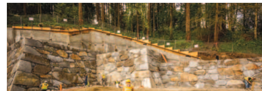
◀ May 2016. The completed Castle Wall.
