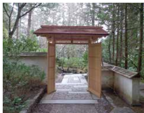
The new gate installed
